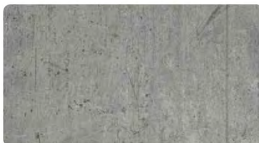
D1038 TO Millennium Concrete
